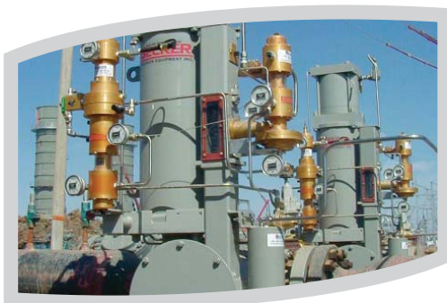
Figure 1 - QTCV-T1 used as primary regulator in power plant
