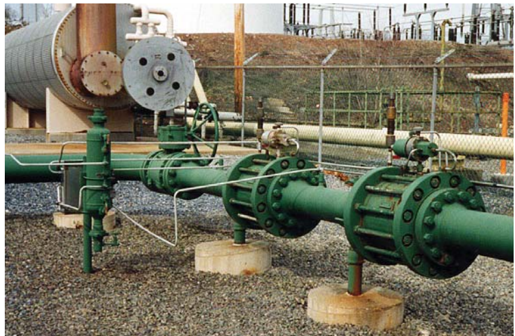
Figure 11.0 - REDQ™ Model 80 regulators in series with REDQ™ Model 820 pilots (superceded by FEP-1000-CH and FEP-1300-CH) configured for downstream pressure control.
