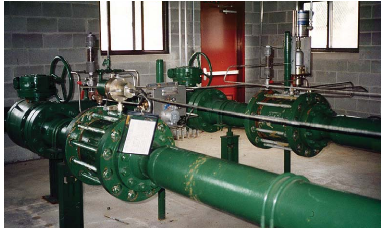
Figure 10.0 - REDQ™ Model 80 regulators in parallel with REDQ™ Model 820 pilots (superceded by FEP-1000-CH and FEP-1300-CH) configured for downstream pressure control.
