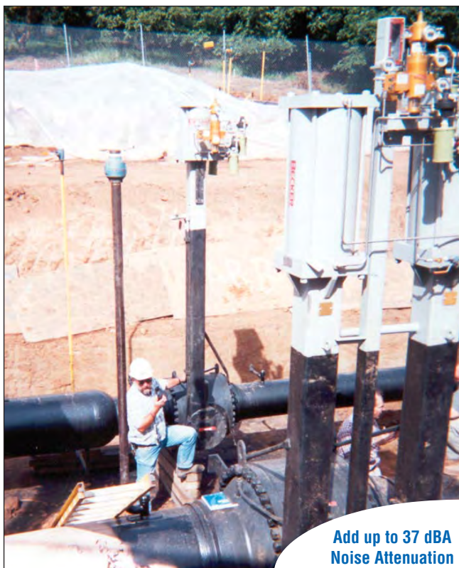
Figure 11 - Installation of Becker Below Ground Regulators (Prior to Backfill)
