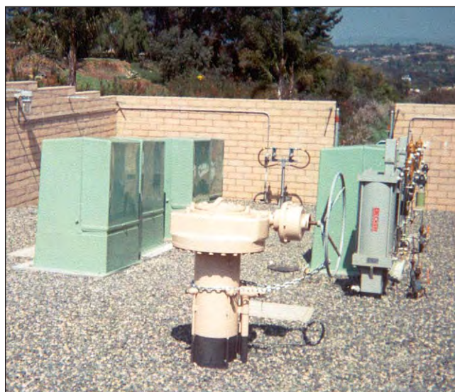
Figure 12 - Installation of Becker Below Ground Regulators (After Backfill)
