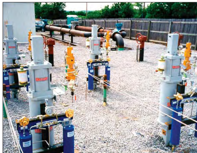
Figure 14 - Installation of Becker Below Ground Regulators (After Backfill)
