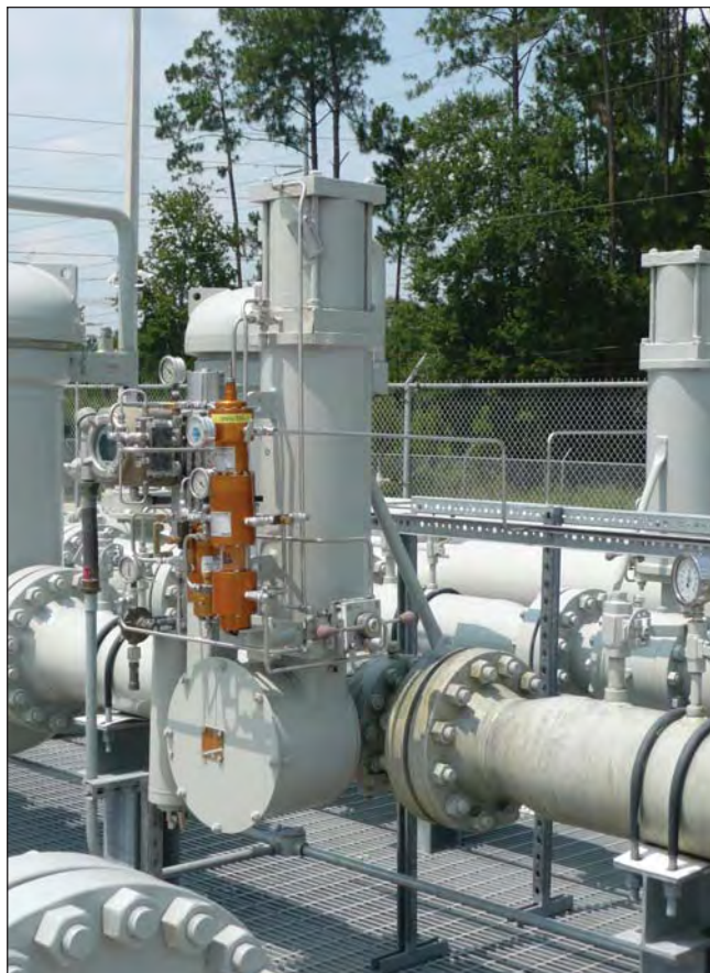
Figure 2 - Model RPSR Rotary Piston Spring Return Actuator Installed in a Power Plant
