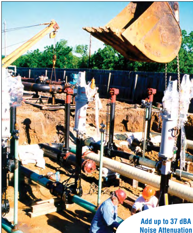
Figure 13 - Installation of Becker Below Ground Regulators (Prior to Backfill)
