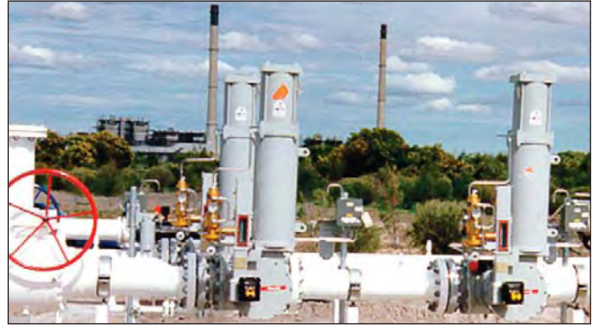
Figure 15 - Becker RPSR Actuated Control Valves in Power Plant
