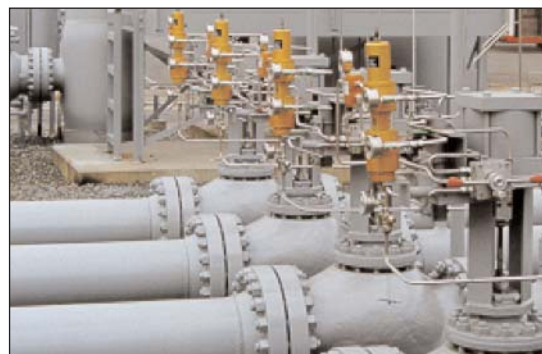
Figure 8 - Becker Model VRP-Pilots on Globe Valve Regulators Becker VRP combined with Becker LPDA Series Actuators used on globe pattern valves are ideal for regulation in LDC systems. Incorporation of the BPS™ feature eliminates all atmospheric emissions.
