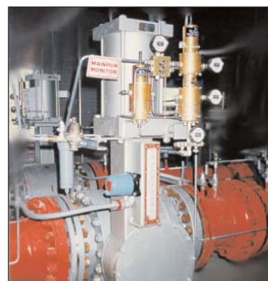
Figure 9 - Becker Model VRP-Pilots on Ball Valve Regs VRP installed on RPDA Series actuator provides reliable overpressure protection in a simple instrumentation package. Note addition of the PS Non-Bleed Sensor eliminates bleed gas when control valve is full-open.
