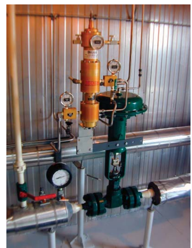
Figure 8 - VRP-SB-CH Retrofit Virtually Eliminates Atmospheric Bleed Gas
