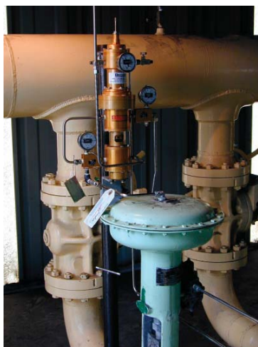
Figure 7 - VRP-SB-CH Retrofit Simplifies Control Instrumentation
