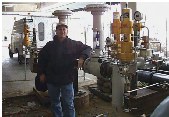
Figure 15.0 - Becker GAP Controller Provides Additional Protection
