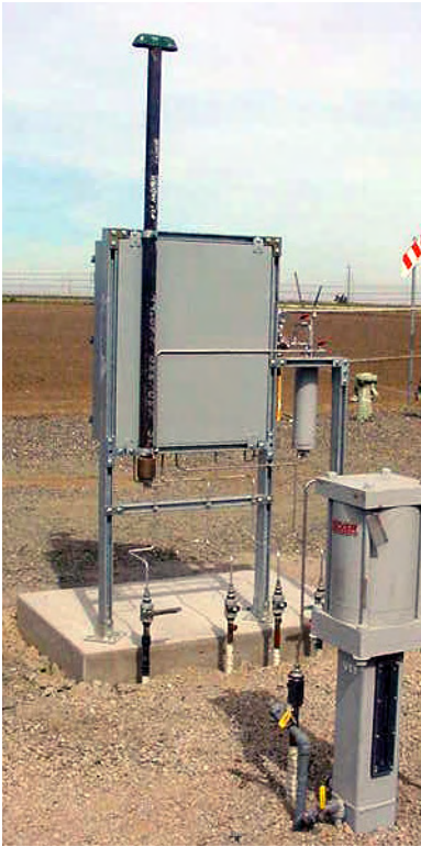
Figure 10.0 - Becker Below Ground Actuated Valve Equipped with VRP-SB-GAP Controller
