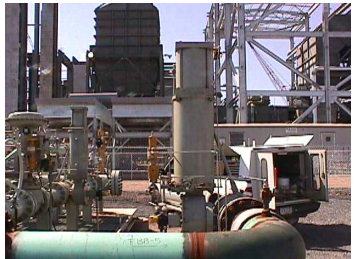
Figure 13.0 - Slam Shut Valve Installed in Natural Gas-Fired Power Plant Fuel Gas Feed
