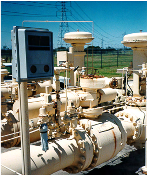
Figure 8.0 - Typical High Bleed Pneumatic "GAP" Controller (Before)
