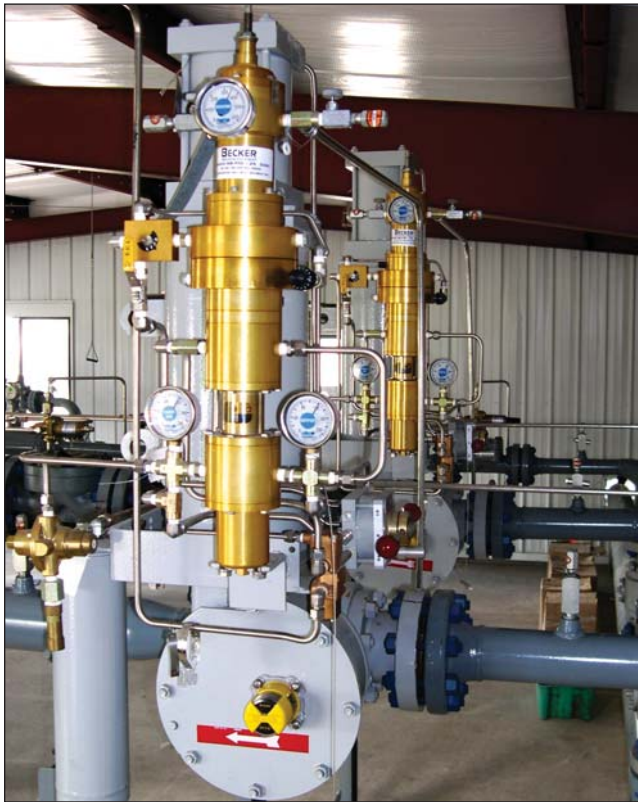
Figure 8 - Becker VRP-SB-PID Installed On A Becker Ball Valve Power Plant Monitor
