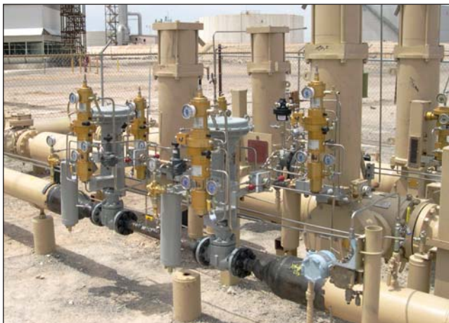
Figure 10 - Becker Designed Combustion Turbine Power Plant Fuel Gas Station
