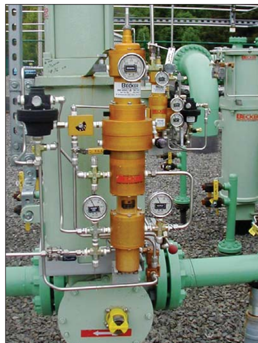
Figure 17 - Becker Ball Valve Power Plant Regulator Utilizing The Becker VRP-SB-PID
