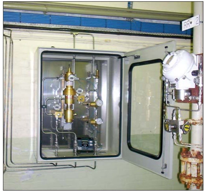
Figure 7 - VRP-SB-PID Retrofit to "Jetstream" Regulator
