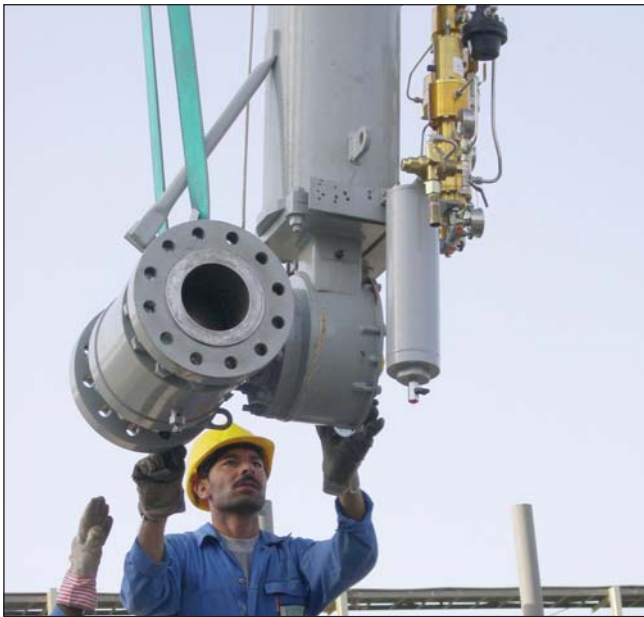
Figure 6 - VRP-SB-PID For Underpressure Protection
